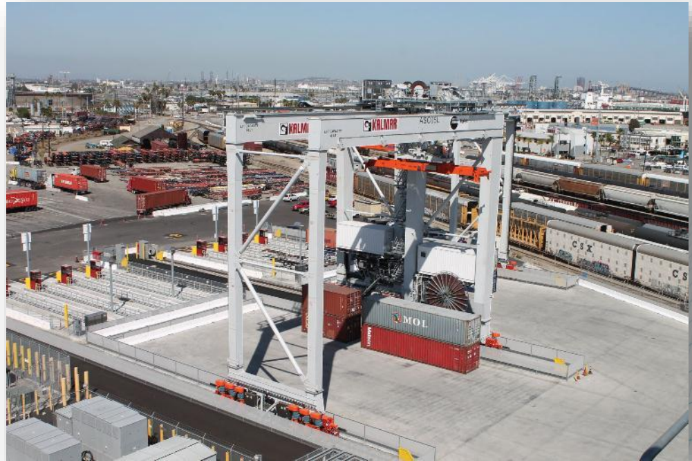
Automated Stacking Crane (ASC)
