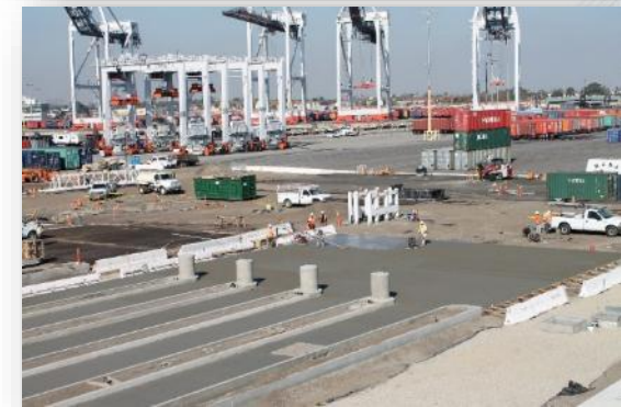
Berth 142-147 Active During Construction
