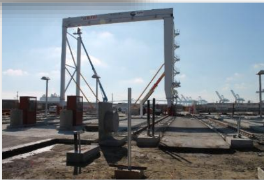
Civil Construction and Crane Equipment Integration
